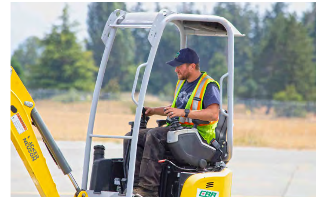
Maintenance/Fuel team member Dave is at the controls for some repairs.
